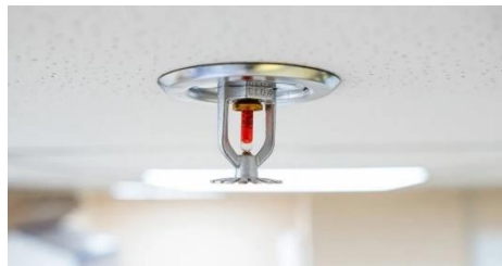
Gambar 5. 22 Fire Sprinkler
