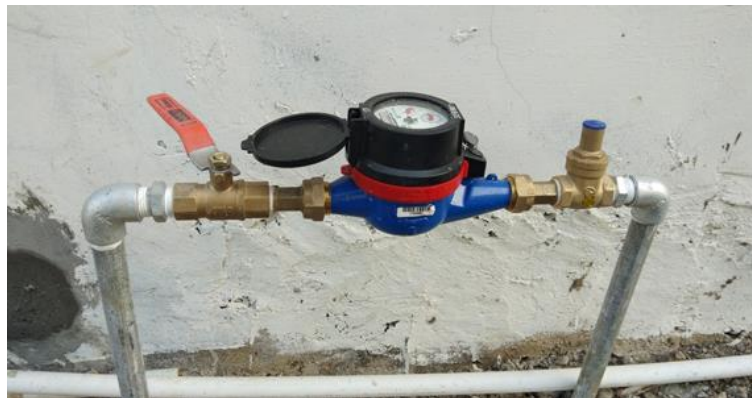
Gambar 3. 1. Meteran air PDAM konvensional [12]
