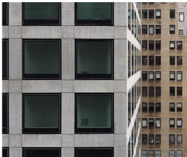
Gambar 15. Fasad 432 Park Avenue.
