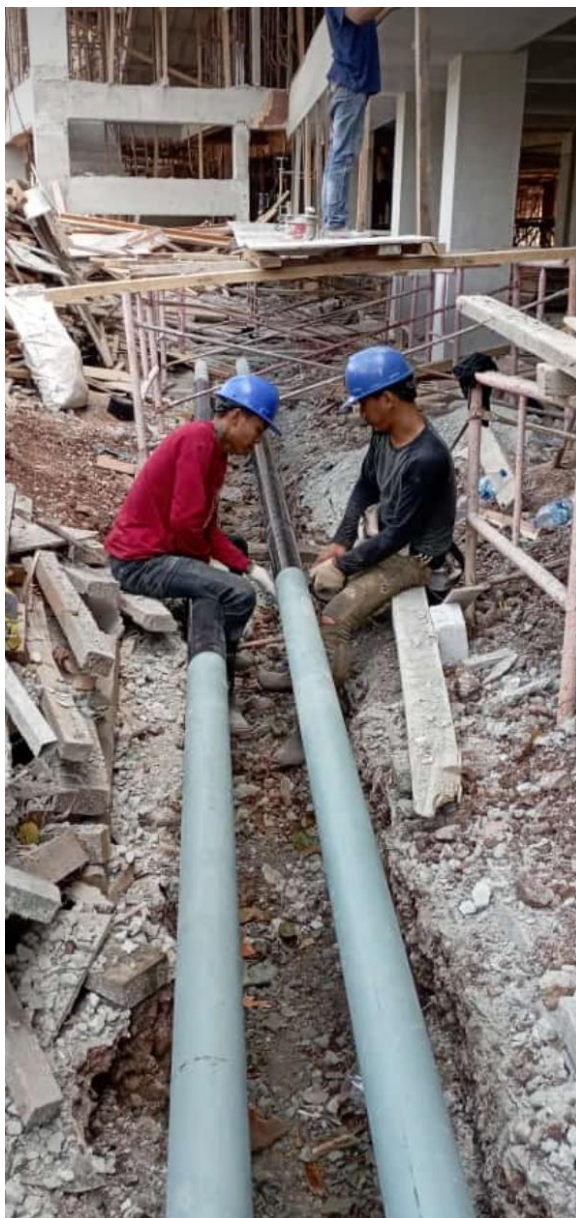
Gambar 4.8 Proses wrapping instalasi pipa hydrant gedung parkir lt dasar as 4-1
